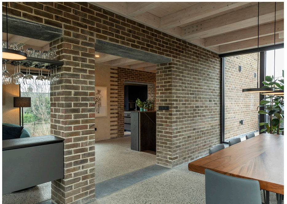
Cross view from the living room
